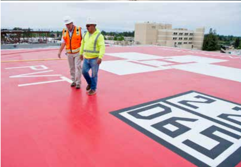
Located behind Washington Hospital, our new parking garage has 648 parking spaces for staff and a heliport on the roof of the structure.
